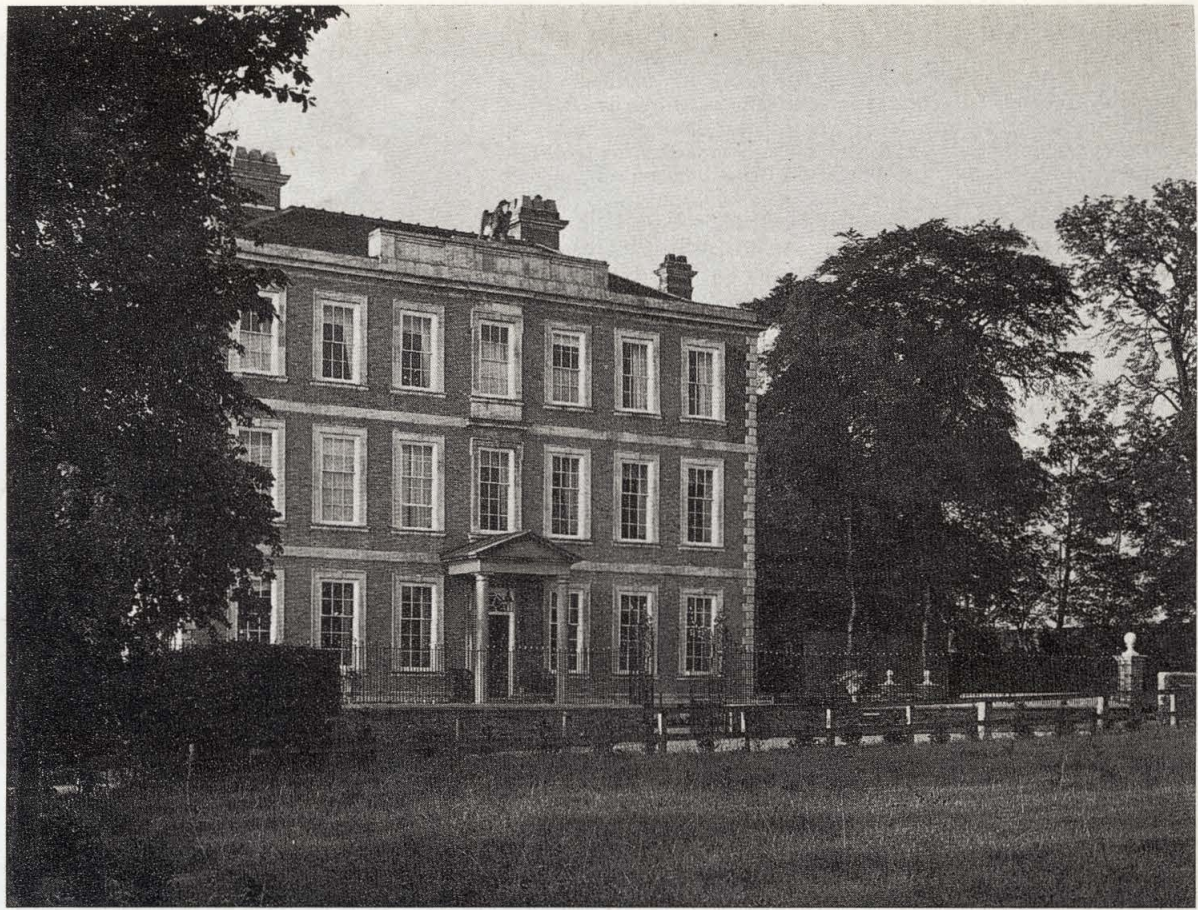
4—THE ENTRANCE FAÇADE. The columned porch was part of the 19th-century alterations
