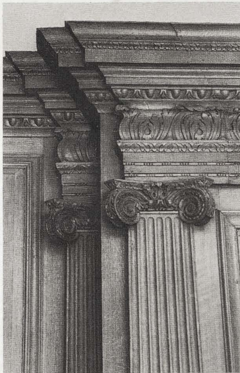
11—A DETAIL OF THE WOODWORK IN THE DINING ROOM. During the recent restoration, layers of paintwork were stripped to reveal the quality of the panelling
