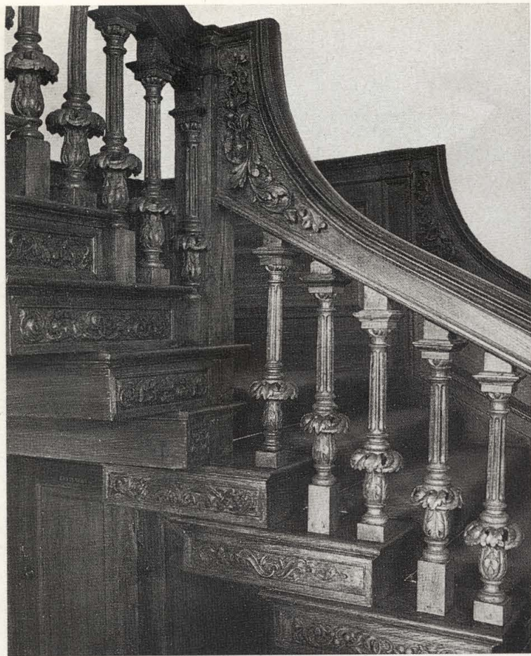
9—A DETAIL OF THE STAIRCASE BALUSTERS
